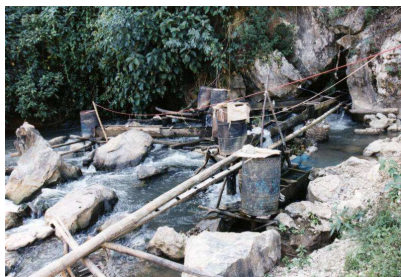
Micro Hydroelectric generation in NW Vietnam village. Set-up involves bamboo and wooden sluices channelling water into oil drums fitted with hand-carved bamboo turbines. Electricity generation was via motorbike alternators. Interestingly, high-tension power lines ran through the middle of the village, but clearly were not used by the villagers.
